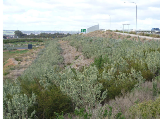
Northern Expressway after the establishment period. Bands of tussock planting have died, leaving large unvegetated areas resulting in weed invasion.
