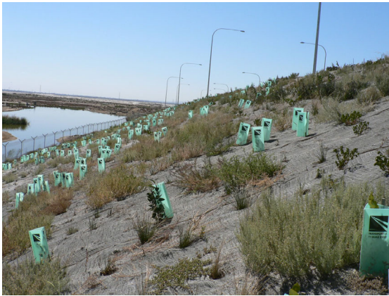
Successful use of thin jute matting to stabilise batter and suppress weeds.
