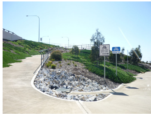
Successful batter planting incorporating trees, low ground covers and a good drainage solution.
