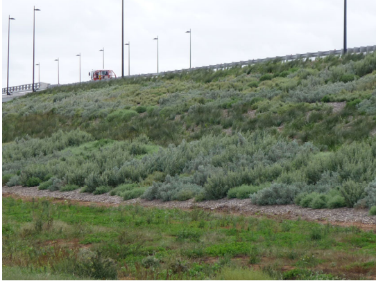
Northern Expressway banded batter planting towards the end of the establishment period.
