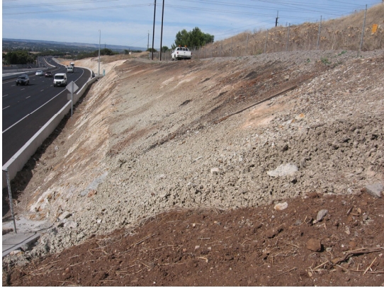
Poorly prepared batter has not been decompacted and will allow minimal moisture infiltration, resulting in a poor landscape outcome.
