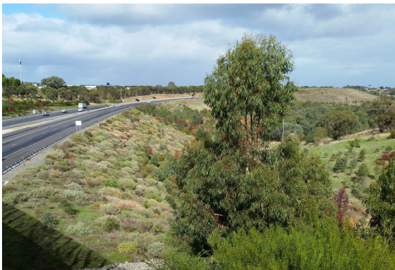
Successful vegetation establishment on a Southern Expressway batter.
